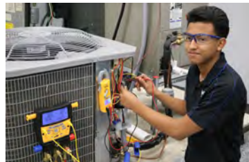
Heating, Ventilation, Air-Conditioning / Refrigeration Approx. 12 mos. | $5,826.95
